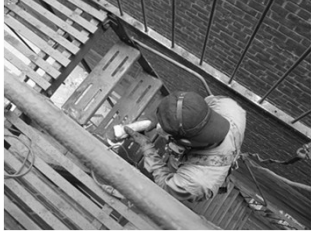
Fire escape repair & load testing
